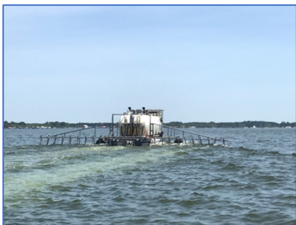
Figure 1. Applying P-binding compounds to a lake.
