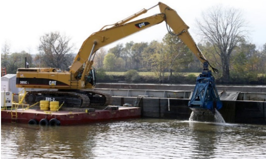
Figure 1. Mechanical dredging on the upper Hudson River.
