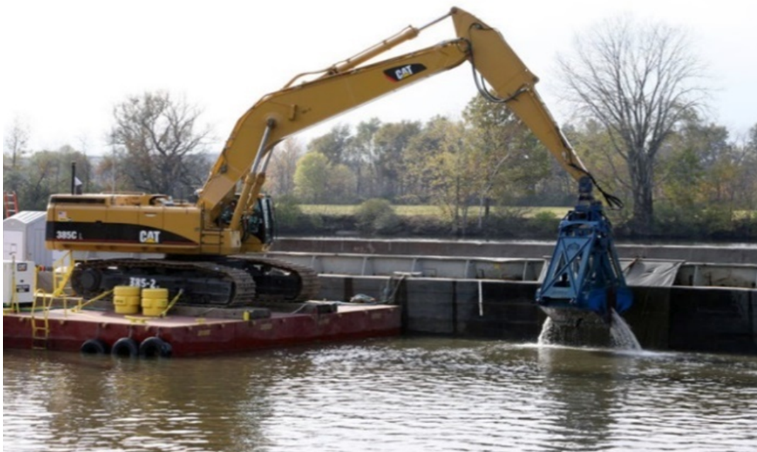
Figure 1. Mechanical dredging on the upper Hudson River.
