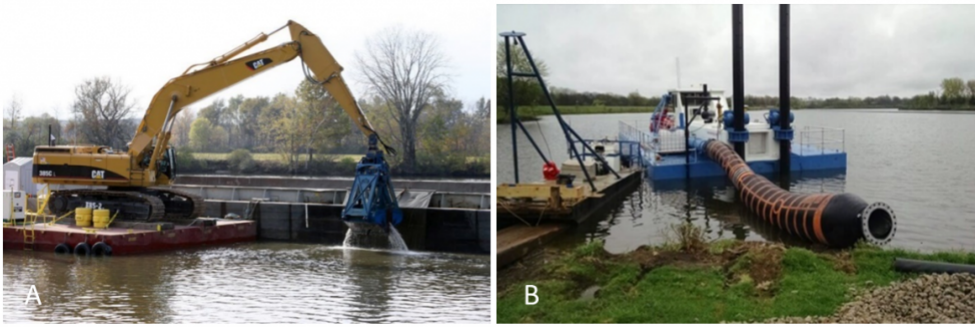
Figure C-3. Mechanical dredging on the upper Hudson River (A) and hydraulic dredging equipment on Easter Lake, IA (B).
